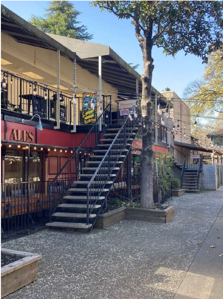
North façade of 217-219 E Street, view facing southwest. ESA, 2024.
