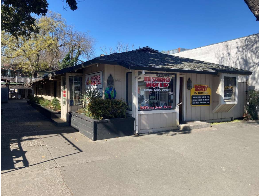
East façade of 223 E Street, view facing northwest. ESA, 2024.
